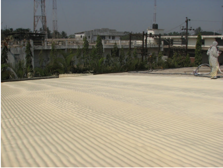
An almost perfect application of sprayfoam roofing
