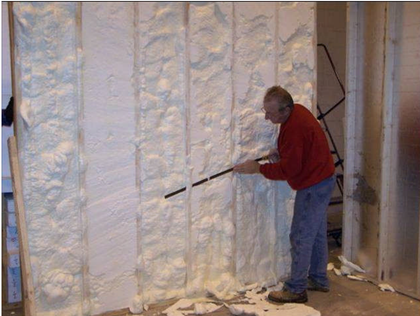
Open cell foam application: Allow at least 20 % waste factor for trimming when Filling stud walls
