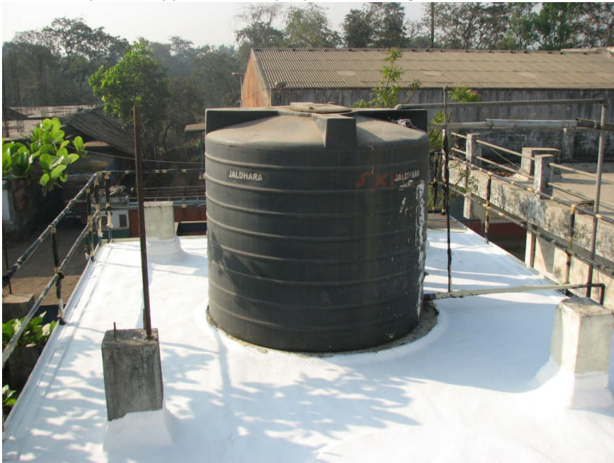
An almost perfect application of sprayfoam roofing
