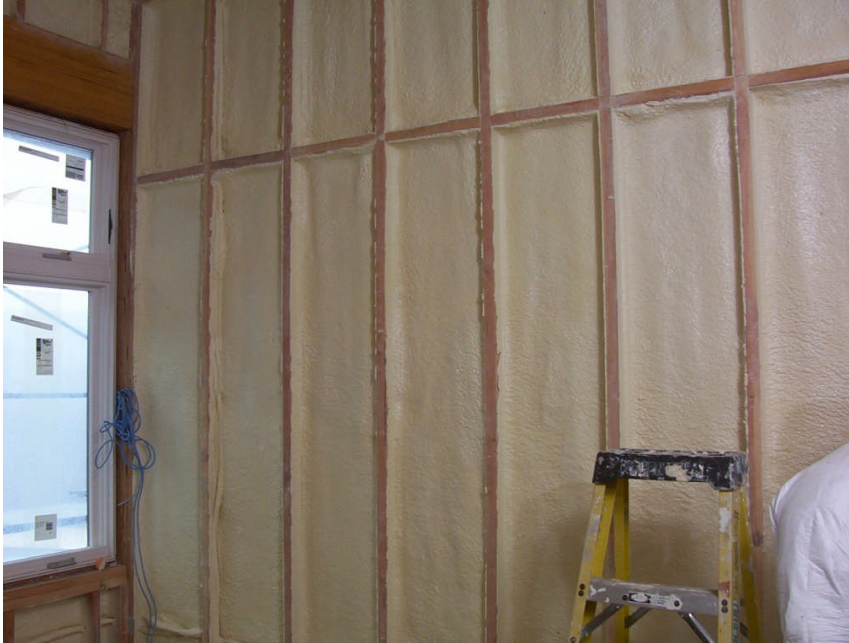
Open cell foam application: Allow at least 20 % waste factor for trimming when Filling stud walls
