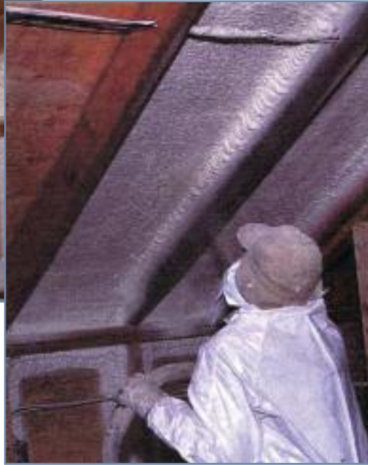
Photos 5 and 6 – Closed-cell foam should be installed in a “picture frame” technique to ensure uniform installation and to enhance adhesion to the studs.
