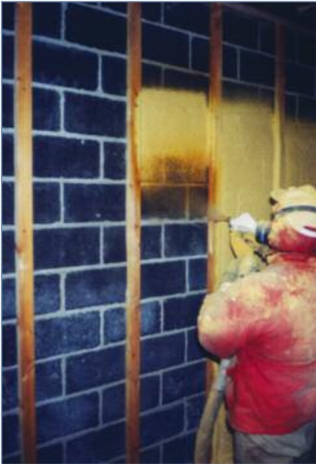
Photos 1 and 2 – ccSPF can be installed between the studs to the thickness desired to provide energy efficiency, thermal comfort, condensation control, and to meet code requirements.
