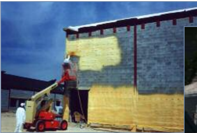
Photos 8 and 9 – ccSPF provides a water-resistant air barrier to the exterior of buildings, reduces thermal bridging, and can enhance the resistance of the structure to high winds and wind-driven debris.
