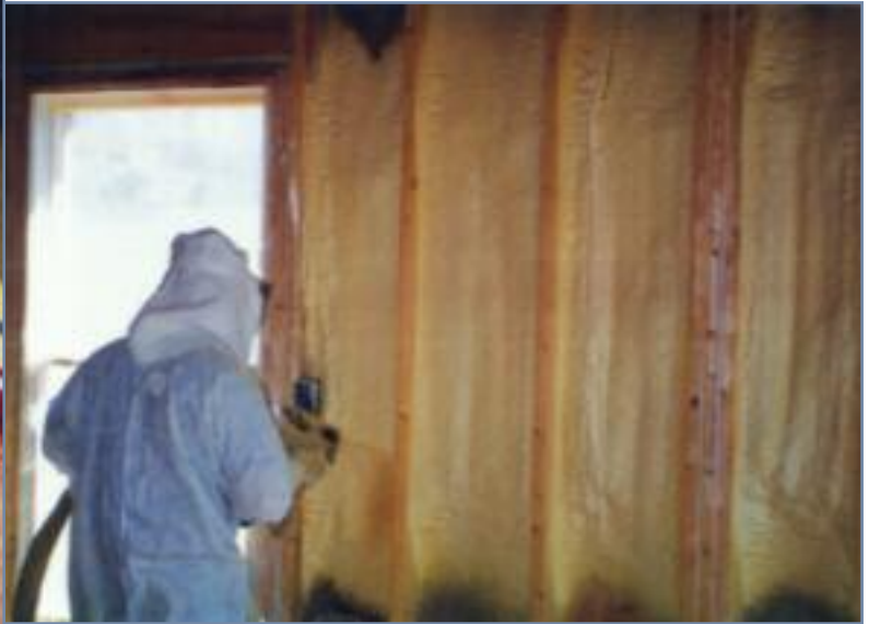
Photos 1 and 2 – ccSPF can be installed between the studs to the thickness desired to provide energy efficiency, thermal comfort, condensation control, and to meet code requirements.
