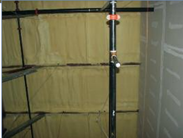
Photos 3 and 4 – Here, ccSPF is installed to the interior of a metal building without studs. This type of application has an added benefit of reducing thermal bridging through the metal beams and columns.
