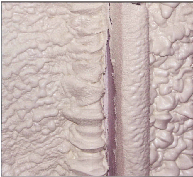
Sprayed polyurethane foam (SPF) shrinkage on wood studs. Different foam plastics rely on different 'ingredients.'
