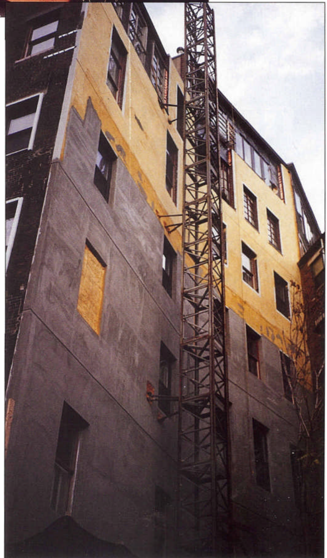
Exterior air barrier application. The Canadian phase-out of HCFC blowing agents need not have a negative effect on building professionals.
