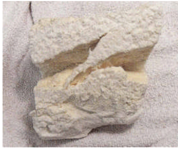
A Cracks, fissures, and voids in closed-cell foam indicate either a poor mix or excessive lift thickness.
